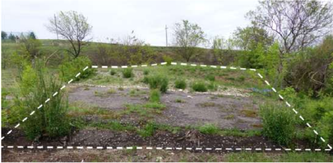
Fig. 6. Surface area of the two vaults, in the foreground the surface of the asphalt layer can be seen and in the background the partly soil covered end of the vaults (width ca. 10 m, length 22 m) [5].
